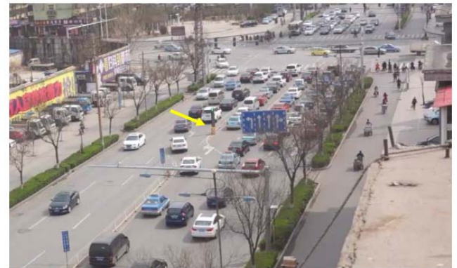
Source: Professor Pan Liu of Southeast University School of Transportation with arrow overlay added by Leidos, Inc. to indicate the presignal location.
