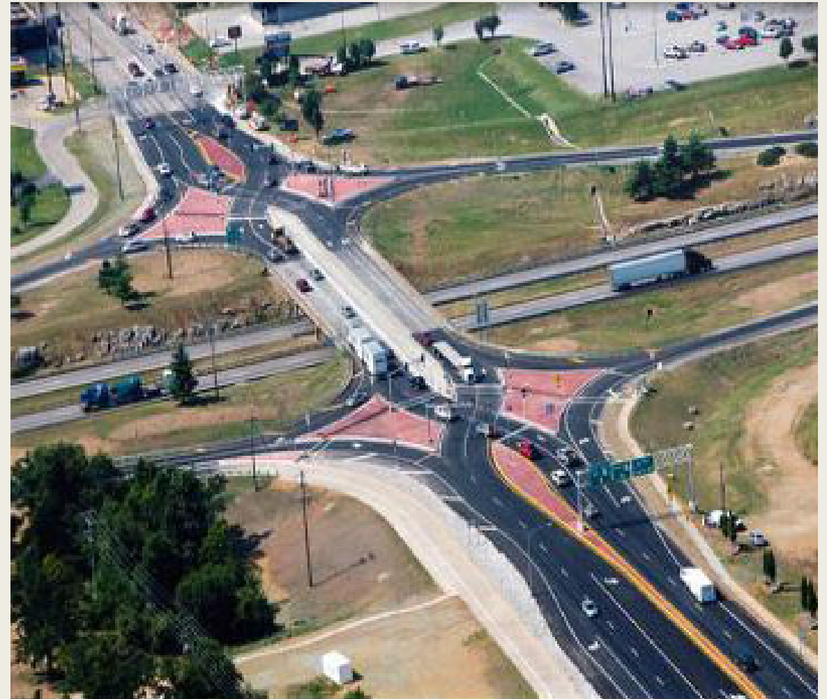
I-44 & Kansas Expressway in Springfield, MO
