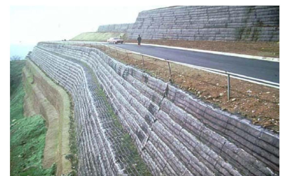
Figure 6 Steeper Roadside That May No Longer Warrant Barrier Protection Source: FHWA http://www.fhwa.dot.gov/engineering/geotech/pubs/nhi10024/nhi10024.pdf
