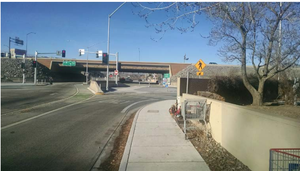
FIGURE 2 – Crossing at I-590 / Moana Lane Northbound On-Ramp with PSD and SSD Issues (Reno, Nevada, Photo: Chlewicki)
