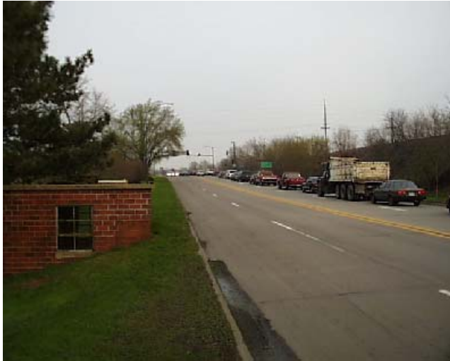
FIGURE 2 Four-lane undivided roadway/intersection operating as a “defacto” three-lane cross section.
